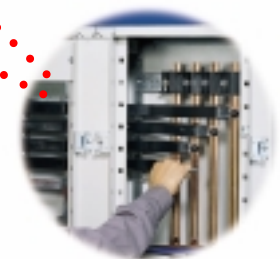
Prefabricated kits for connection between circuit-breakers and busbars
